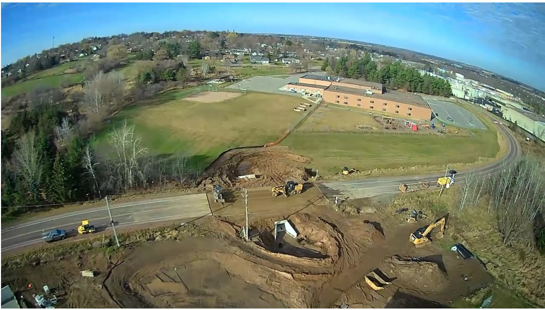
4 th Street Pedestrian Path, CTH NN Tunnel Construction, November 24'
