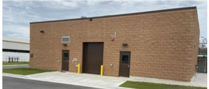
Blower and chemical building
