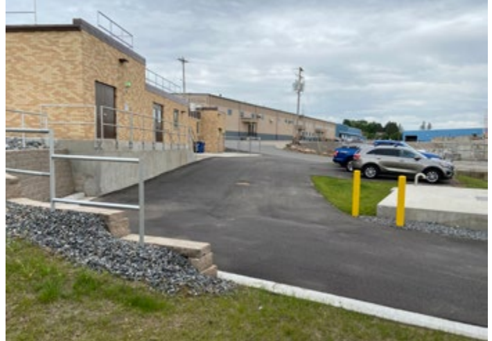
New roadway, parking area, and retaining wall
