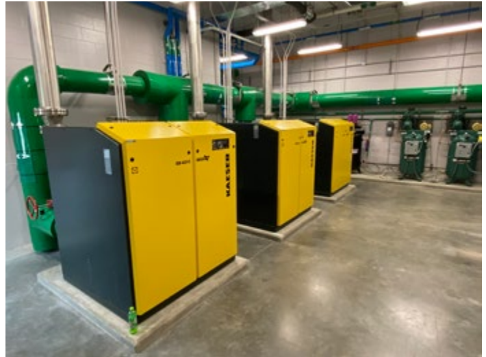
Positive displacement blowers
