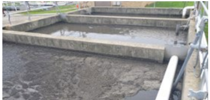
BPR tanks before upgrade
